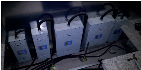
The MPE filters in situ at JIAT
